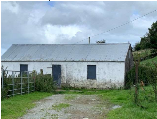
5. Single storey outbuilding
