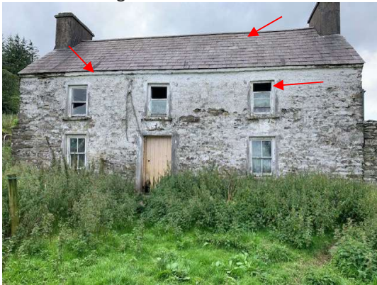
3. Derelict dwelling indicating potential access points via soffit, ridge tiles and gaps in roof tiles and open window.
